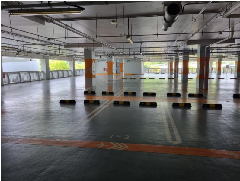
Car park spaces 151, 152 and 153
